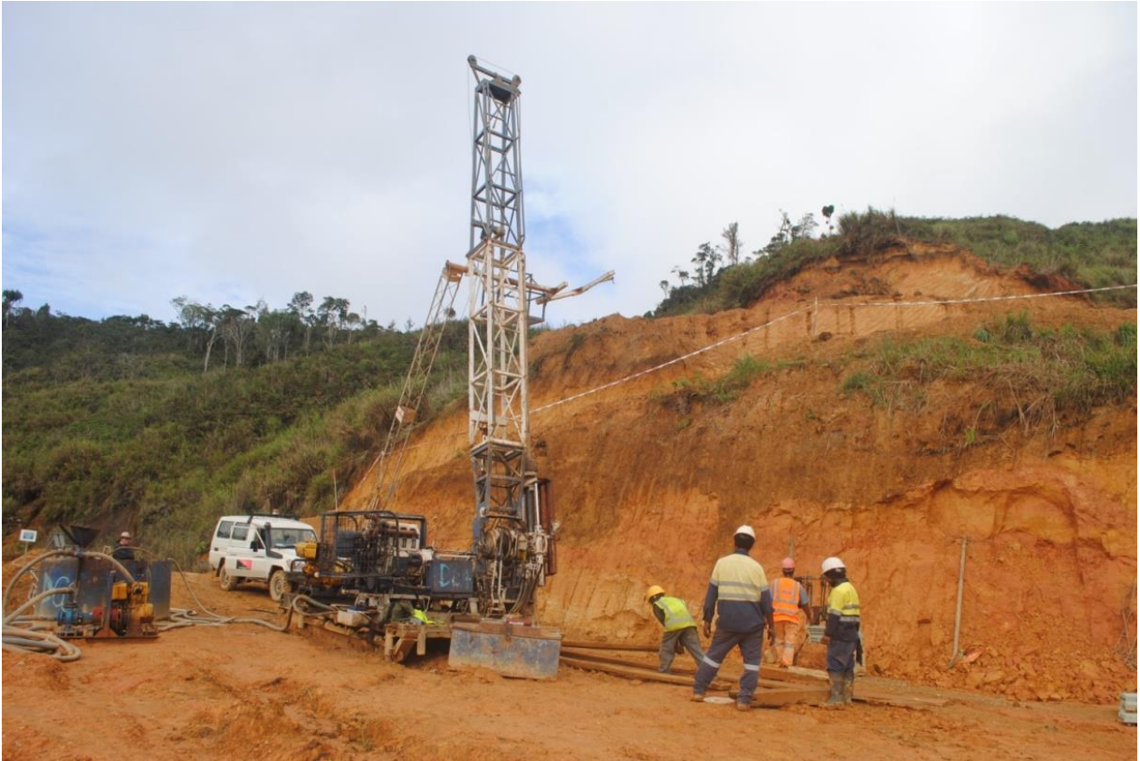
Figure2: Niuminco drill rig and team drilling the Enterprise vein system
